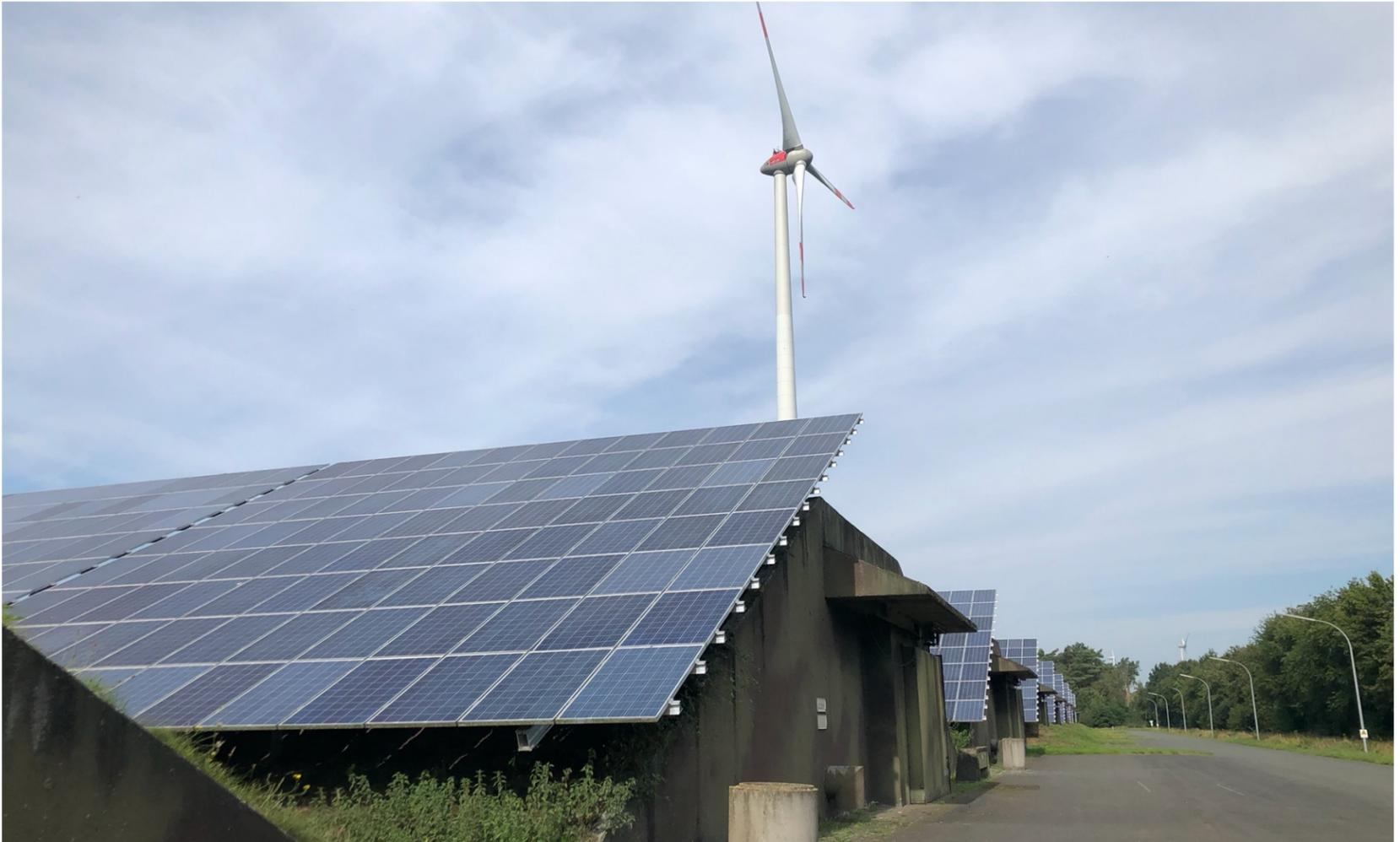
The old military munitions bunkers at the Bioenergie Park have been repurposed to support and cool the solar arrays.
